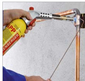
Brazing in gas installation
