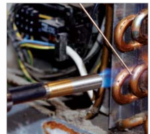
Hard soldering in refrigeration and climate control
