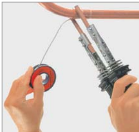
Warming up of the soldering point without open flame
